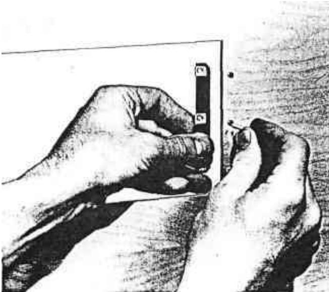
Insert the screws in the center holes of the cabinet panel ("B" holes on the template) and tighten. The screw head should pull into the wood slightly. (Use two  $\frac{3}{4}$  inch long screws for panels under  $\frac{1}{2}$  inch, or two VA inch long screws for panels  $\frac{1}{2}$  inch thick and larger.)
